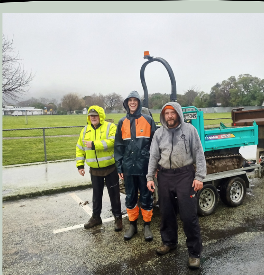
Building the skills track in the rain
